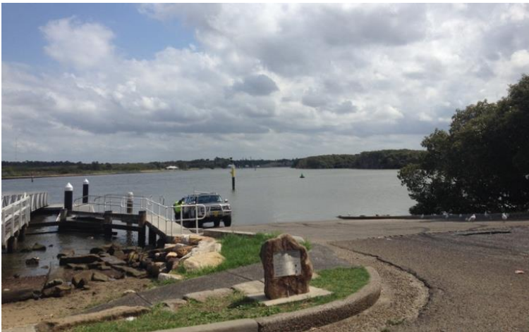
Figure 20: Existing boat ramp and wharf (Source: AJC)
