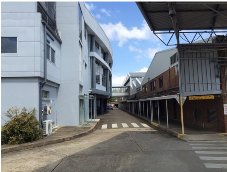
Figure 29: Existing industrial buildings on Site (Source: MWC)
