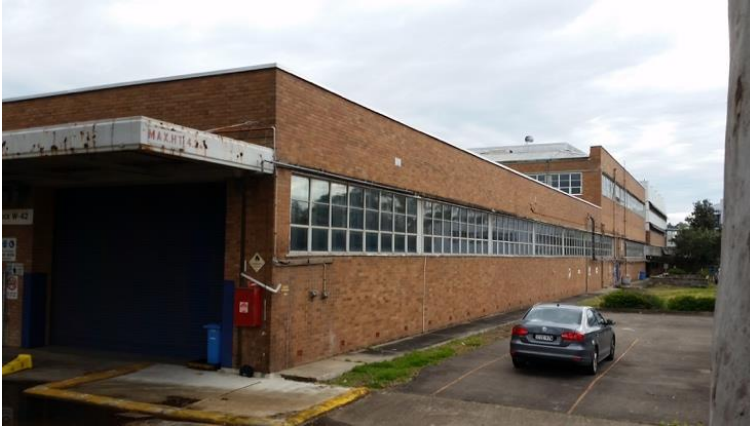
Figure 31: Existing buildings Hope Street (Source: AJC)
