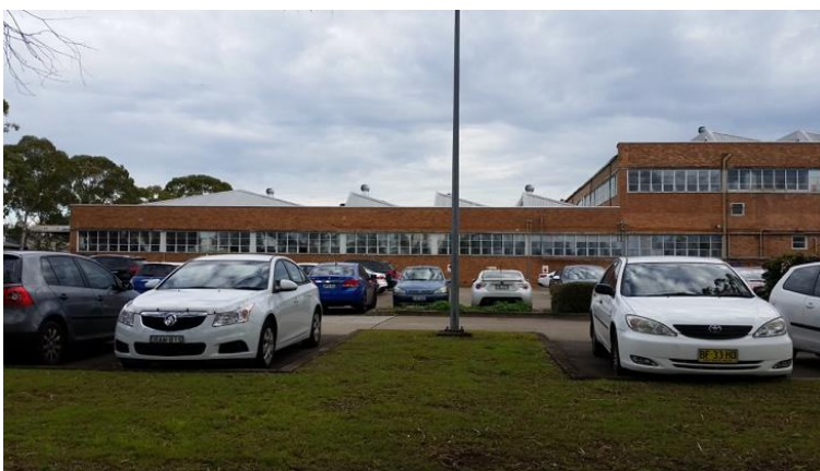
Figure 30: Existing industrial buildings at Wharf Rd (Source: AJC)
