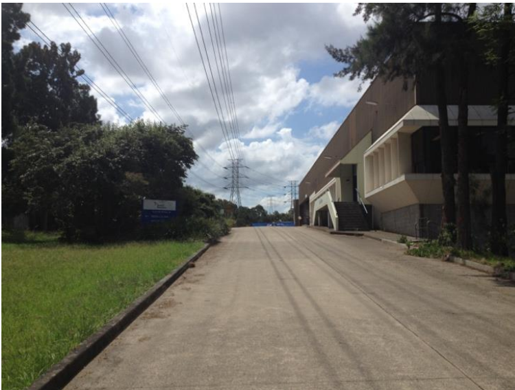
Figure 24: Transmission lines on Site looking north (Source: AJC)
