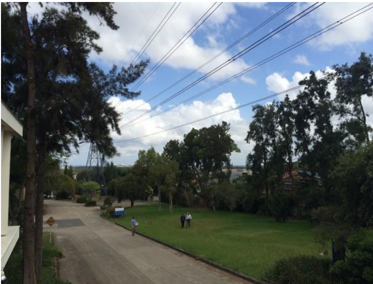
Figure 23: Transmission lines on Site looking south (Source: AJC)
